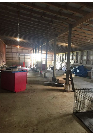
The humble beginnings of where we are working to place the forge. The previous owner left it in quite a mess and disrepair.
